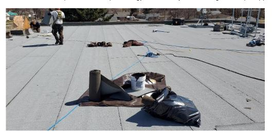
2.02 Existing bagging stripping will be fastened with screws and plates before the recap stripping is installed.
