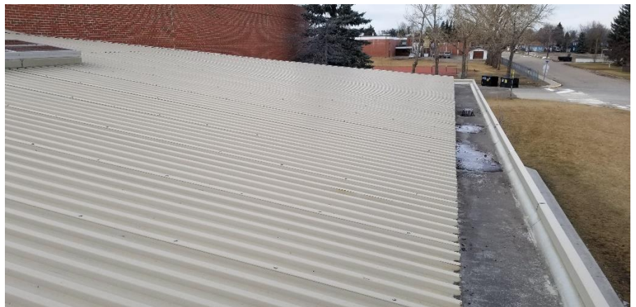
62) Gutters around the steep-slope roof should be cleaned.
