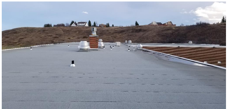
32) The roof is SBs and for the most part is in good shape; some minor repairs are required.
