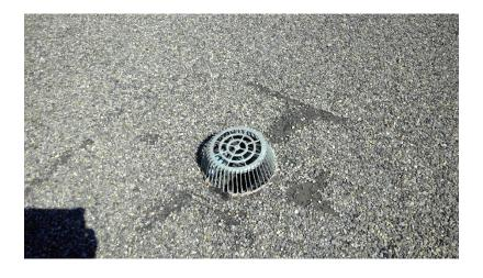
5) The Bay – Exposed felts around the drain.
