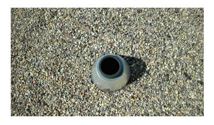
North Central Mall - Area A Tall cone with no pipe should be capped to keep the water out of the building.
