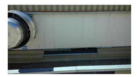
24) South Central Mall - Area I Proper cladding should be installed on this detail, wind driven rain can get in the building.
