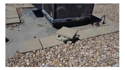
34) Milestones – Displaced pavers and gravel should be replaced.
