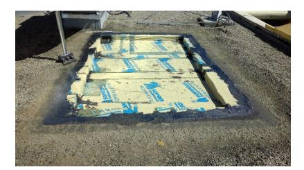
20) South Central Mall - Area G, temporary seal for unit install is not adequate for longer term. This should only be used for an overnight seal with little rain expected.
