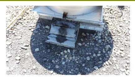
33) Milestones – This grease collector is not working properly and allowing grease onto the roof. This could damage the roof over time.
